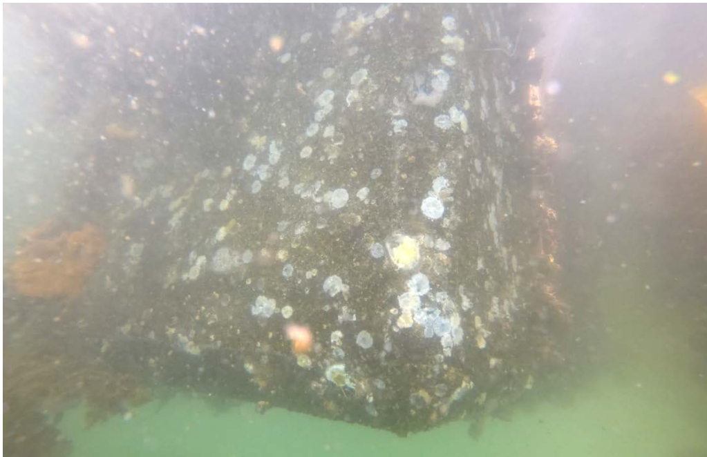
PHOTO No. 8: Concrete Float, Near Pile No. 10 - Note the well defined corners of the concrete pontoon, with no evidence of any cracking, spalling, or rust bleeding visible. No supplemental floatation was noted during our inspection, and the sampling of inspected floats were found to be floating level with good freeboard.
