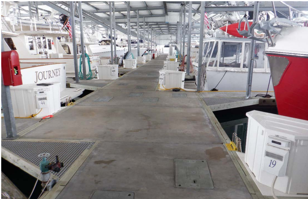
PHOTO No. 4: Marina Float, Main Access, Looking North - Note the overall good condition of the concrete pontoons which are floating level and with good freeboard. Also note the overall good condition of the timber wales securing the individual pontoons together.
