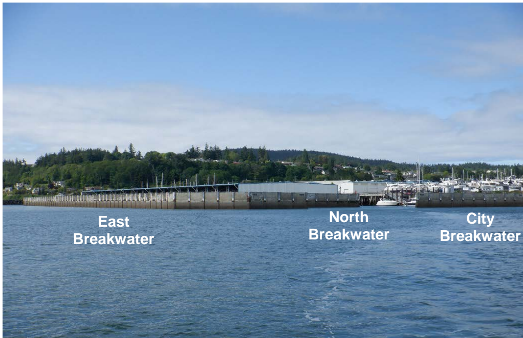
PHOTO No. 1: Fidalgo Marina, Looking Southwest - The marina moorage consists primarily of covered slips constructed with concrete floats that are secured in place by prestressed concrete piles. The marina is protected by a steel pile supported concrete panel breakwater.
