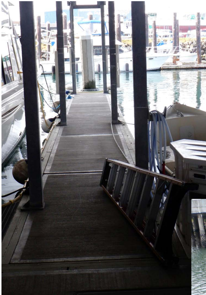
PHOTO No. 5: Float Anchor Pile No. 54, Looking West - Note the overall good condition of the prestressed pile and the individual concrete pontoons which make up the floats. Also note the pontoons are level with good freeboard.
