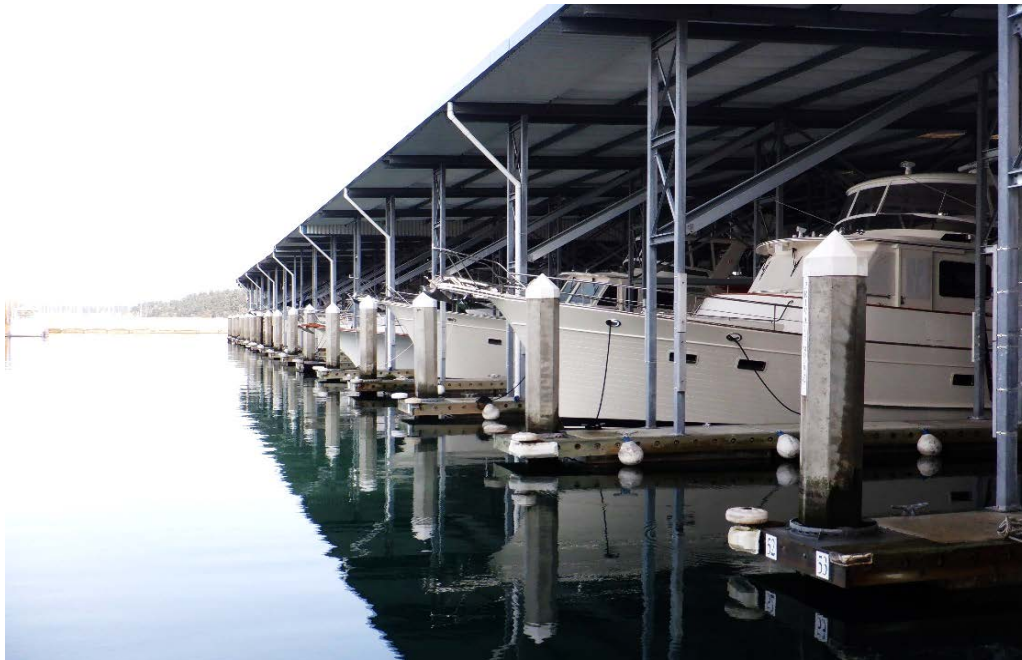
PHOTO No. 2: Marina Moorages, West Edge, Looking North - Note the overall good condition of the prestressed concrete float anchor piles, as well as the steel column and roof support system which bears directly on the floats.
