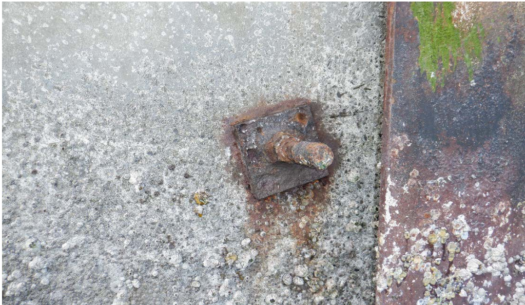
PHOTO No. 16: Breakwater, Exterior Face, Typical Condition - Close up of connection bolt, plate washer and nut shown in Photo No.15 above. Note the moderate to heavy corrosive section loss visible on the hardware. This condition was found to be typical of many of the bolted connections located in the intertidal and submerged zones.
