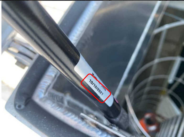
Photograph 8: View of a sticker on the roof hatch dated October 10 th , 2021.
