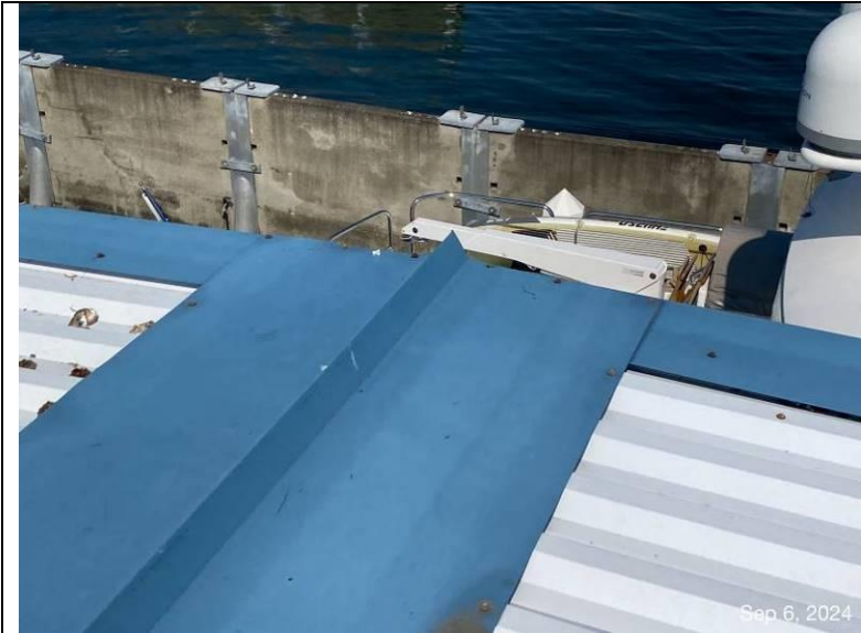
Photograph 25: View of the ridge flashing lapping onto the rake flashings.
