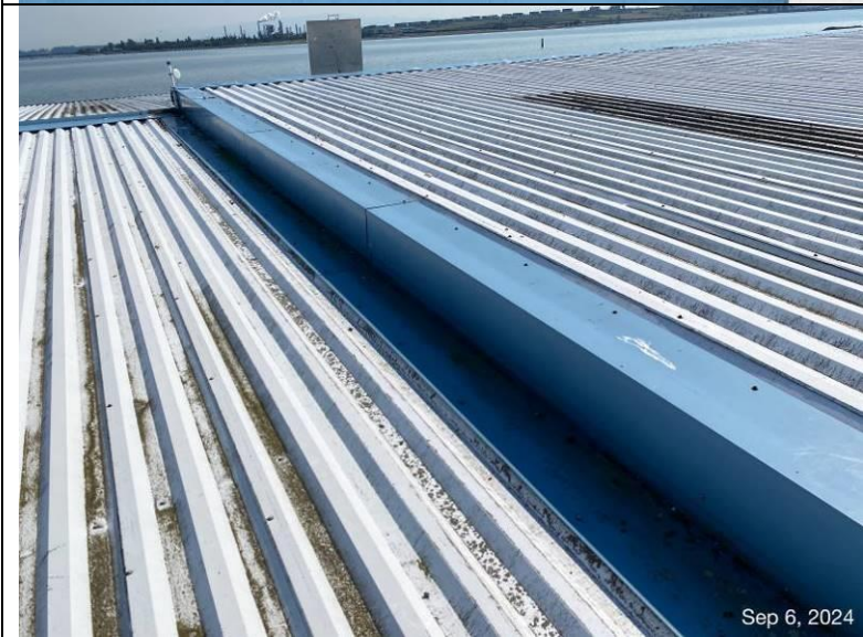
Photograph 27: View of transition flashings at the roof plane changes.
