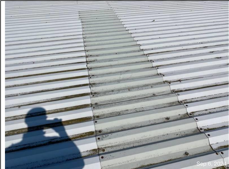
Photograph 52: Alternative view of supplemental roof panels.
