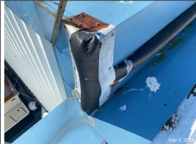
Photograph 34: View of the vertical-to-horizontal transition of the expansion joint.
