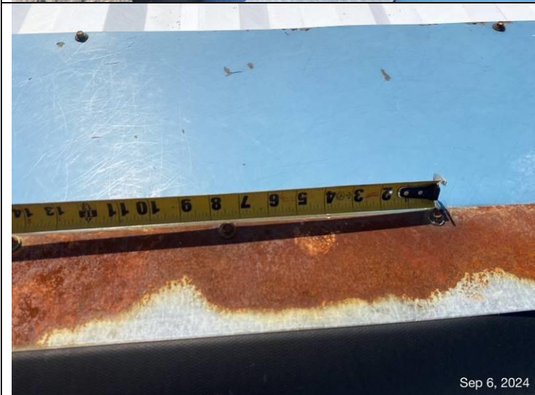
Photograph 39: Expansion joints flanges secured to the sheet metal flashings at approximately 8-inches on-center.
