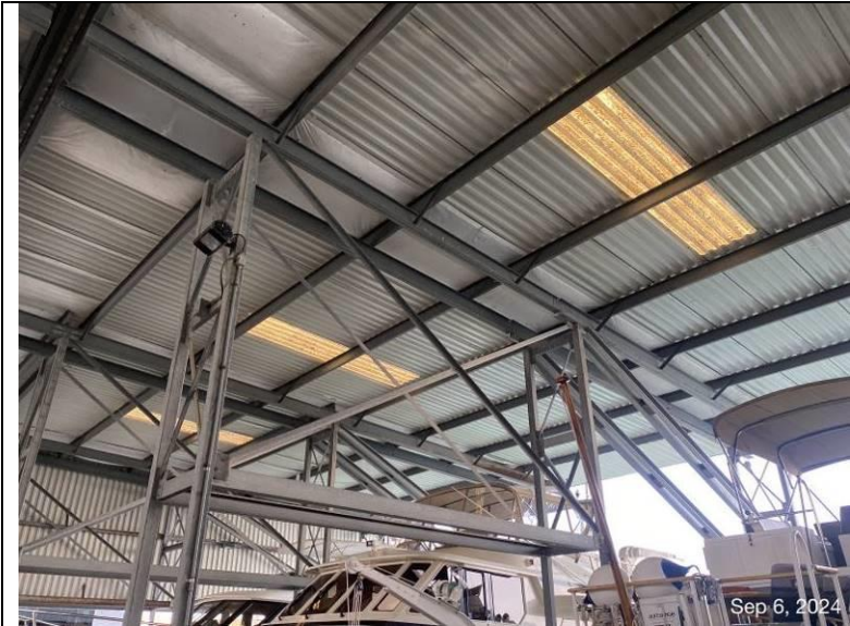
Photograph 10: View of the translucent roof panels from the underside. Note areas where the condensate blanket has been removed.
