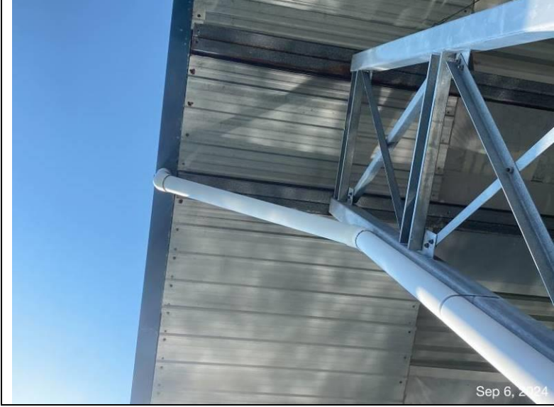
Photograph 21: View of the downspout and prefinished metal soffit panels.
