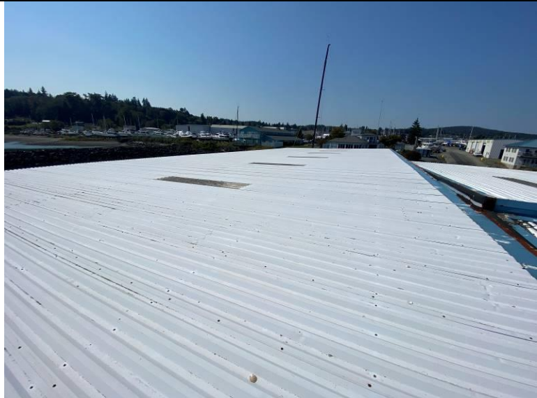
Photograph 3: Overview of the south roof, looking southwest.
