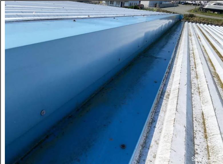
Photograph 28: View of the roof-to-wall flashing tucking under the rake flashing.
