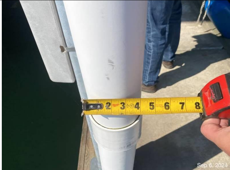
Photograph 22: View of the downspout measuring at 4-inches in diameter.
