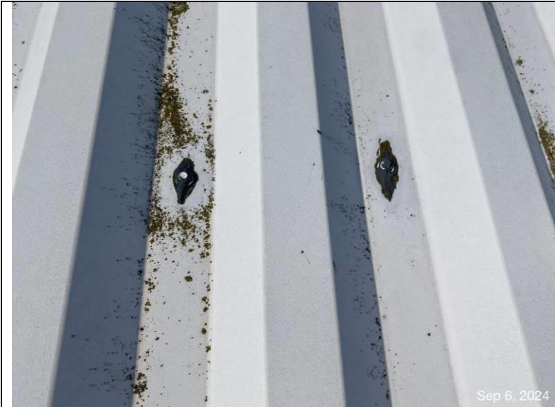
Photograph 13: Fasteners in the field of the roof sealed with sealant.
